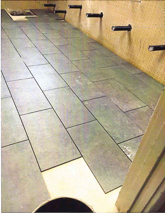
Installation of new tile in the Boys Restroom
